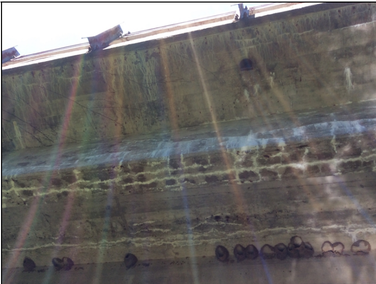
Efflor map cracking span #1 girder #4
